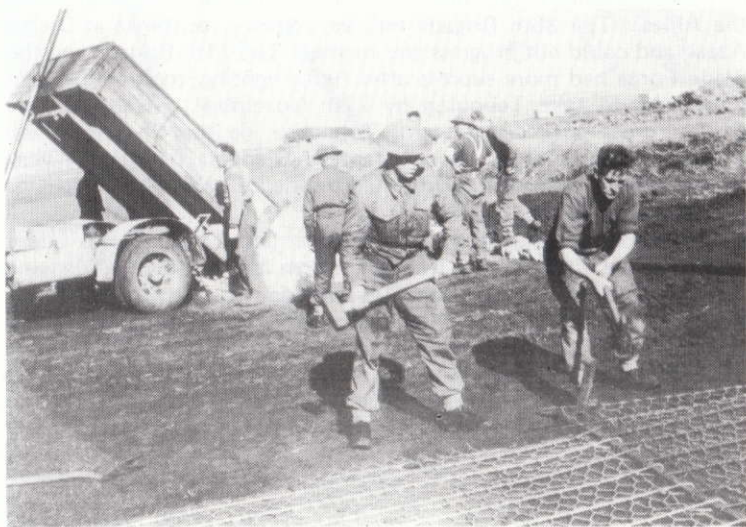
Laying the foundation of the runway and fixing the Somerfeld track.
